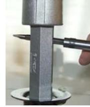
J. At the cut end of the Tub Shoe (#8), slide a 1 3/8" Slip Joint Nut (#6) onto the tube with the threads (grooved end) facing away from the tub. (Fig. 8)
