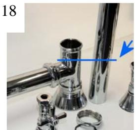
B. With the tube next to the Tub Tee (#7) measure and mark the farthest point the tube will fit inside the Tub Tee. See the blue line on Fig. 18 and Fig. 19.
