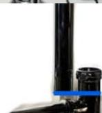
C. Remove the Overflow Head/Tubing Assembly from the overflow drain hole by unscrewing the Face Plate Screw. Using the tubing cutter cut the Overflow Tube where you marked it in step B. (Fig. 20)
