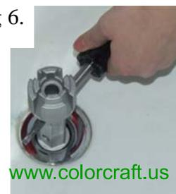
I. Using the P.O. Tool/ Tub Shoe Remover tighten to hand plus 1/4 turn. (Fig. 7) Remove the excess plumber's putty that will ooze out.
